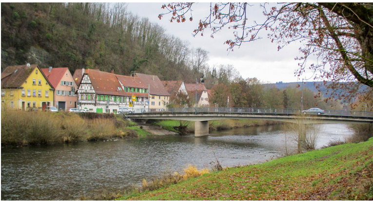
Herrenwaagbrücke in Mühlacker
