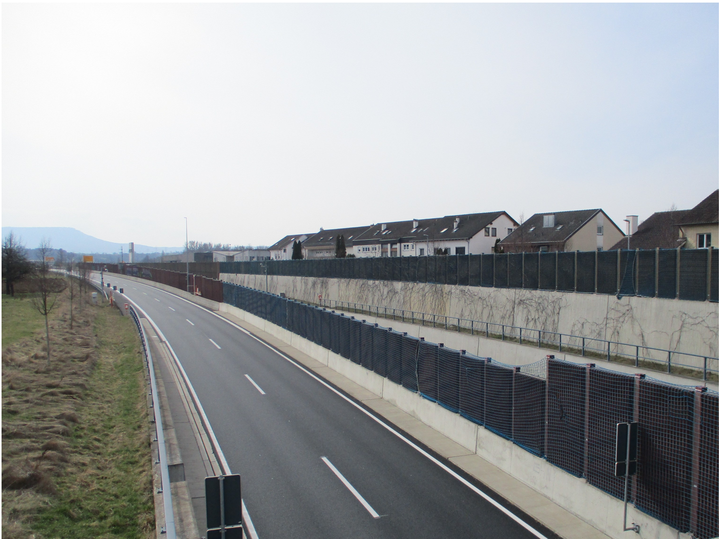
B 27, Dußlinger Tunnel
