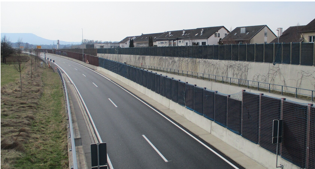
B 27, Dußlinger Tunnel
